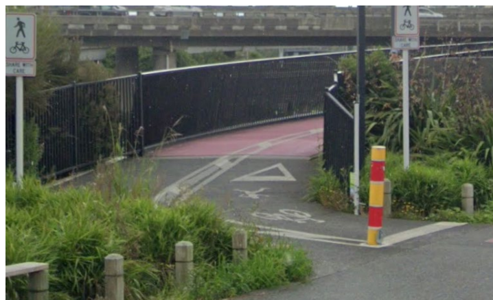
Figure 29: Existing poor visibility around inside corner of The Lightpath (Google, 2023)
