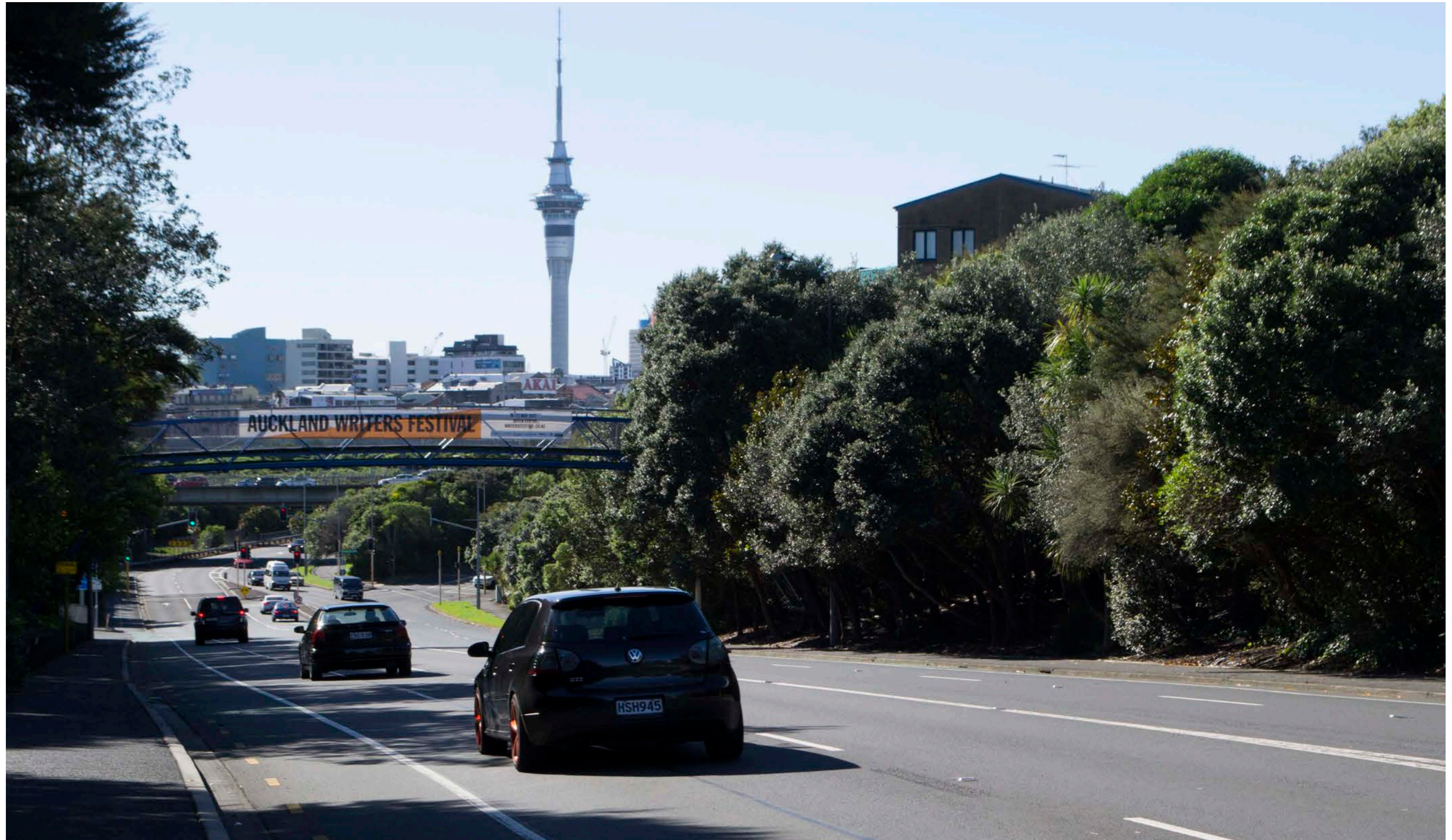
Figure 73 Existing Perspective: Looking north along Ian McKinnon Drive near Haslett Street from the west side kerb.
