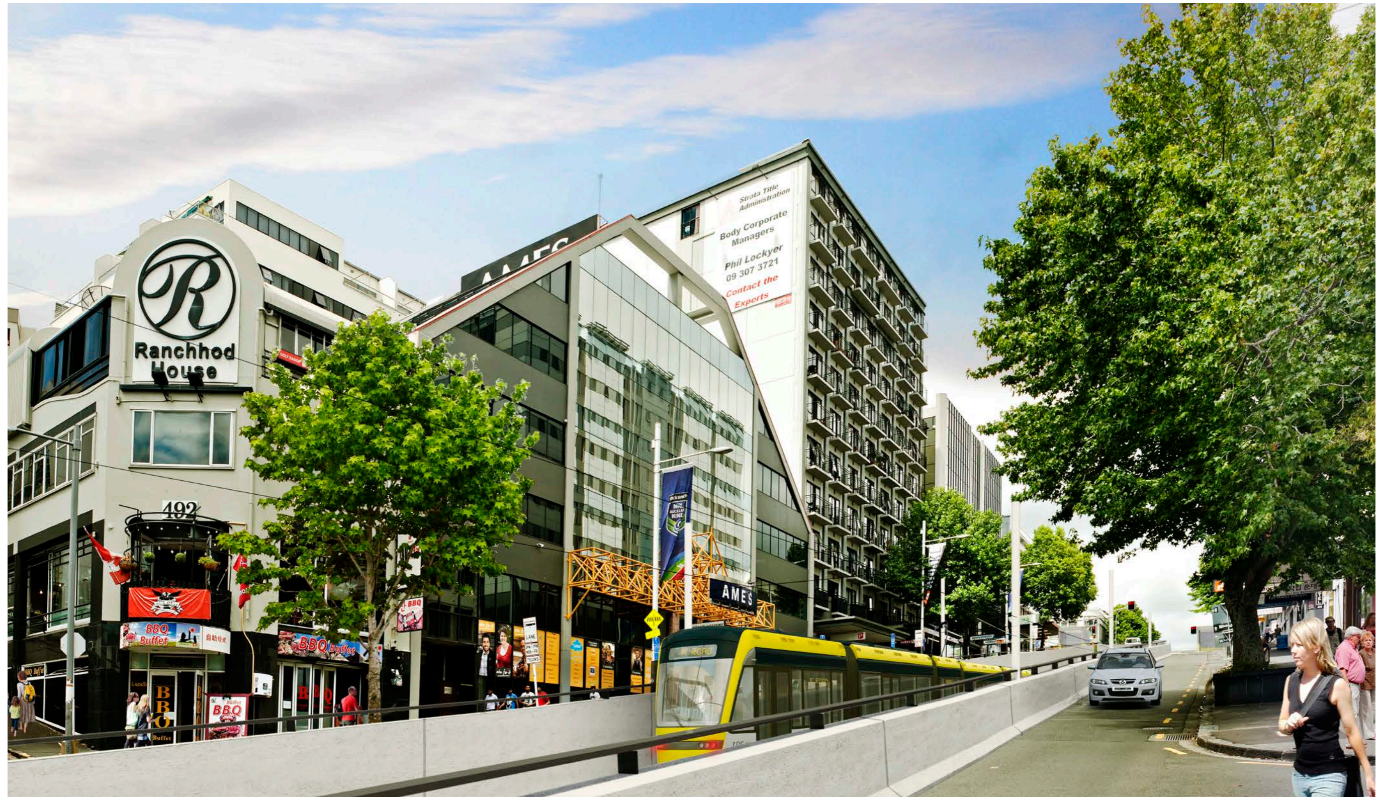
Figure 58 Proposed Perspective: Queen Street looking south east towards Karangahape Road with proposed LRV underpass extending south under Karangahape Road showing indicative underpass architectural treatments and traffic safety barriers.
